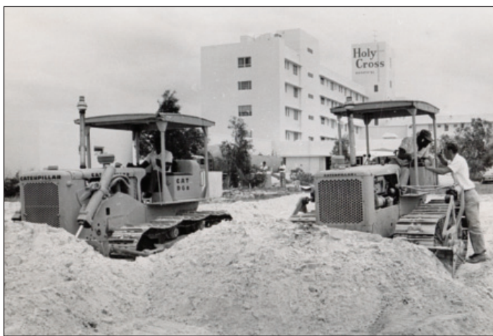
Construction taking place at Holy Cross Health in the mid 1950s, capturing the early development of the hospital
